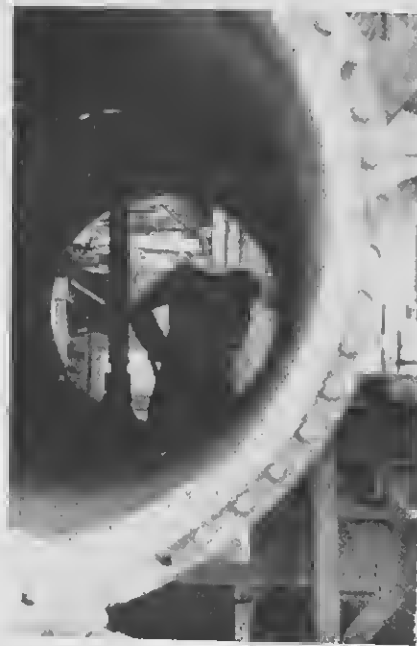
Viewed through the length of an exchanger shell, this workman is using a chipping hammer to clean the inside. He is working at the battlefield (7).
